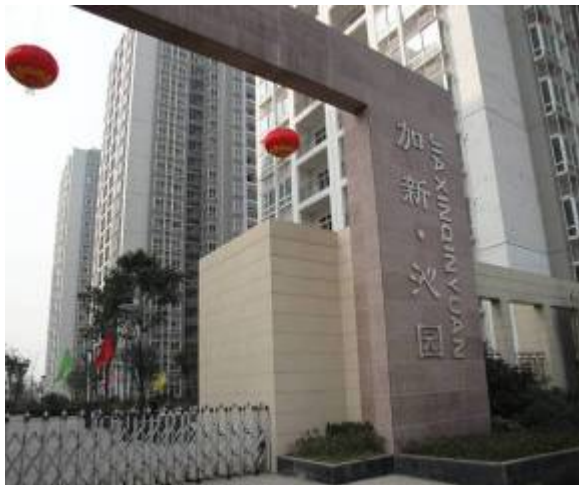
图：已建成的重庆加新·沁园智能小区 Smart community in Chongqing
