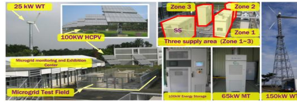
100 kW Autonomous Micro-grid Demonstration System
